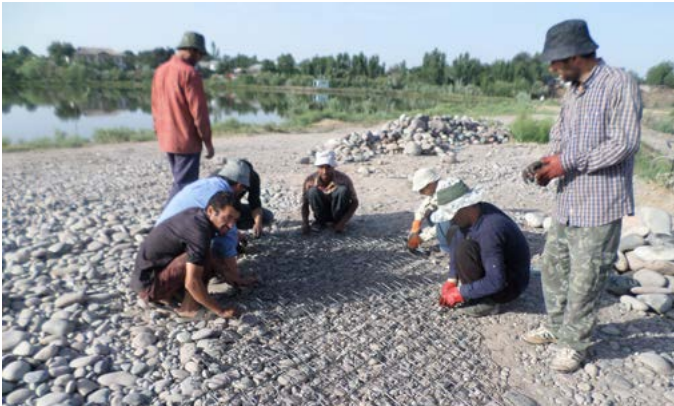
Riverbank reinforcement works during the exercises
