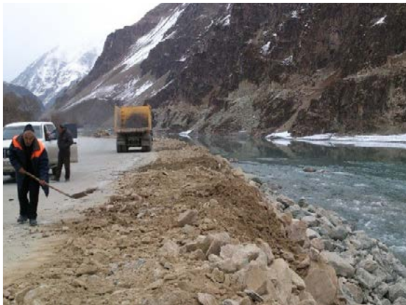
Road rehabilitation in the Darvoz district
