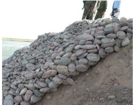
Riverbank reinforcement works during the exercises
