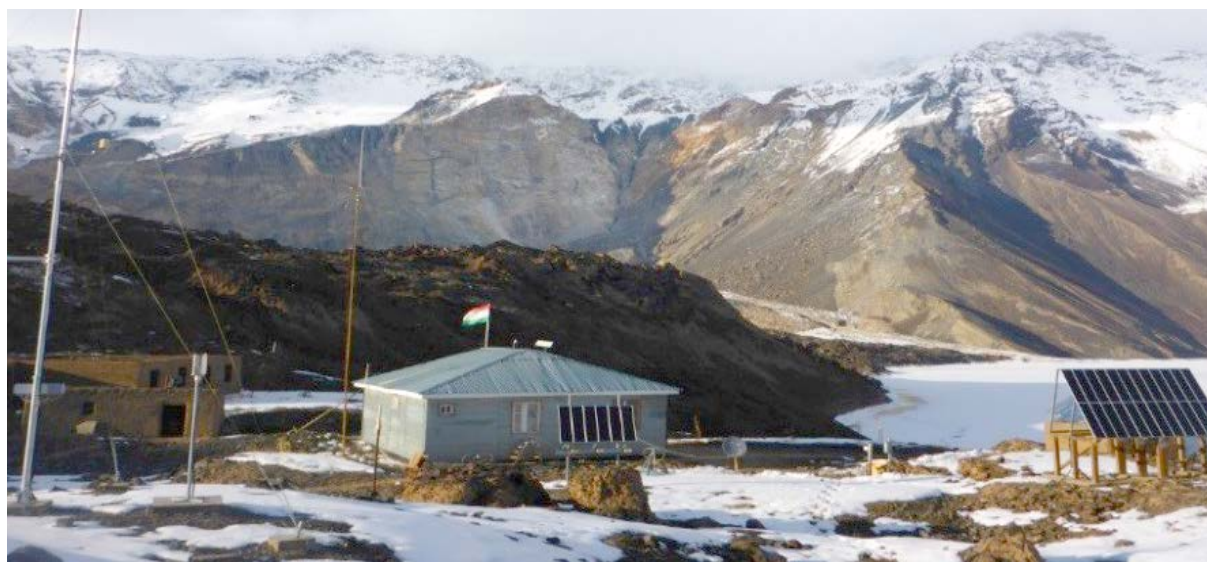
CoES Control Point at the Usoy Dam of the Sarez Lake
